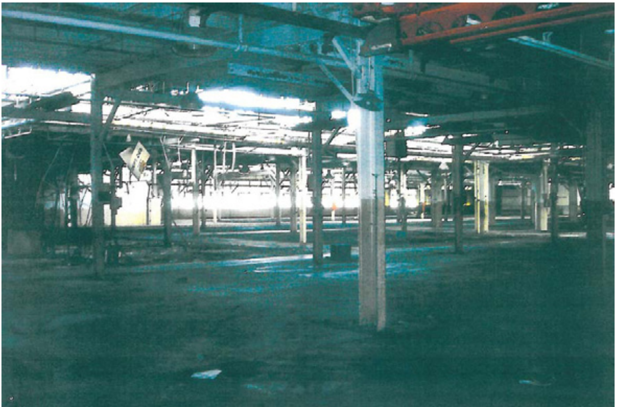
Figure 4: Interior view of the Hercules Motor Company high bay space
