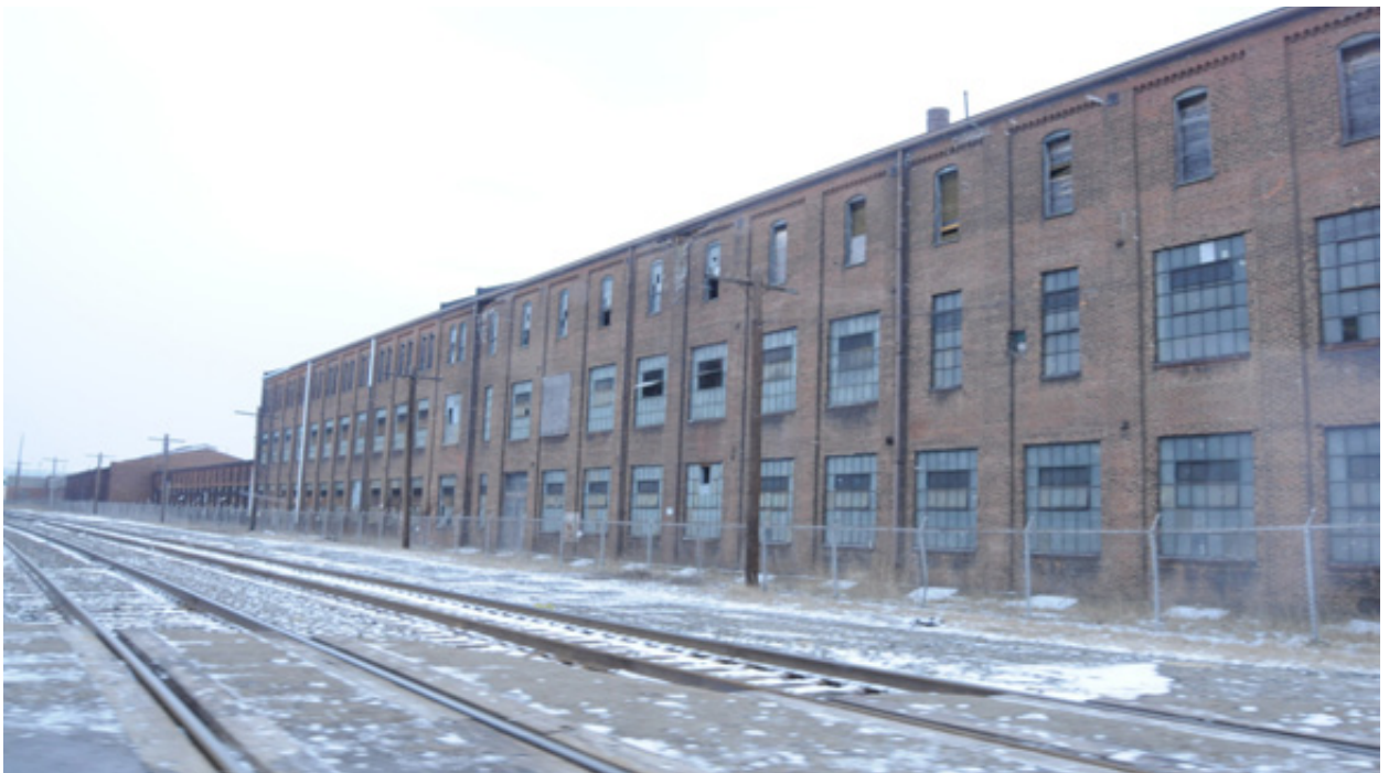
Figure 12: Existing view of Hercules Complex taken from the rail yard to the north of the site, view looking south
