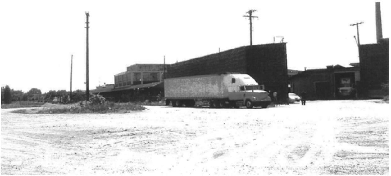
Figure 6: Existing view of Hercules site taken from east entrance
