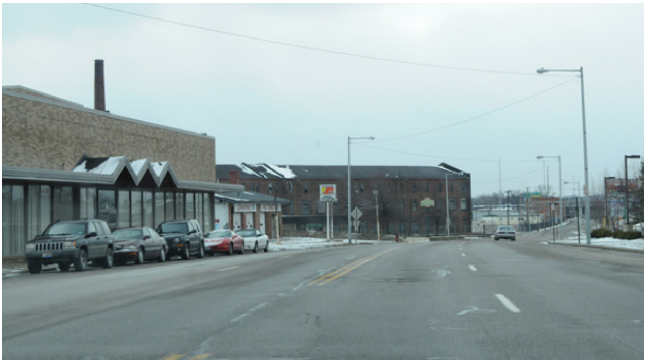
Figure 16: View of Hercules Complex and surrounding context from Market Avenue travelling south toward Highway 30
